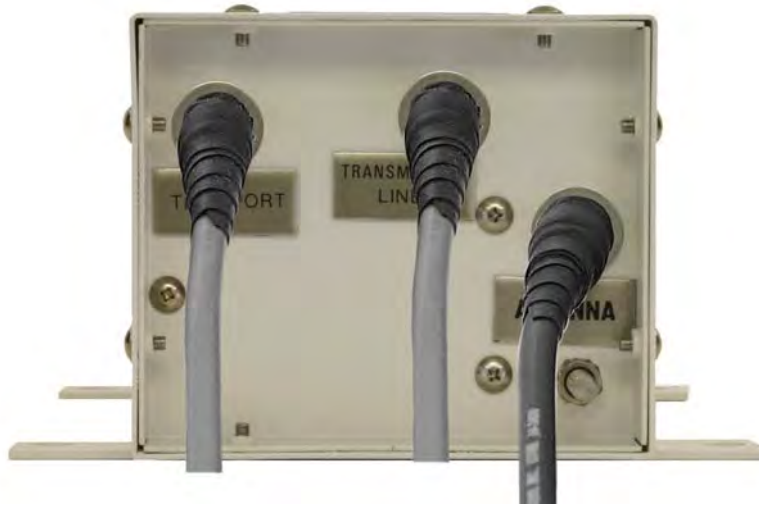
Figure 12: Application of rubber splicing tape. NOTE: Additional waterproofing protection can be realized by covering the rubber tape with either "Scotch Kote" or Vinyl plastic Electrical tape ("Scotch" brand 33+).
